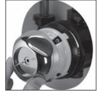
14 Turn on the supplies and check for any leaks upstream of the valve. Slowly open the control and check for leaks downstream of the valve. If all is sound, turn off the on/off knob fully, turn off the supplies and remove the on/off knob.
