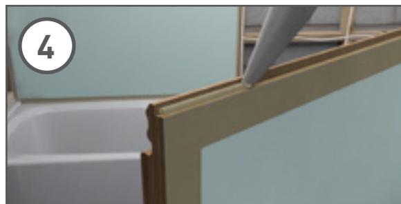
Apply masking tape to the two meeting edges of the decorative face to protect the laminate face. Apply a narrow bead (2-3mm) of silicone sealant to the front shoulder of the tongue.
