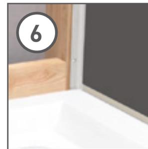
6 Apply high grab adhesive to the reverse of the Multipanel® angle into the first profile and push firmly against the wall.
