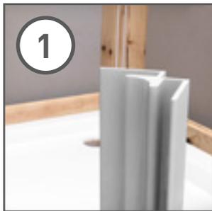
1 The first profile, which normally starts with an Internal Corner or End Cap, should be fixed to the wall or end grounds with countersunk screws, or adhesive and a bead of silicone sealant applied to the channel
