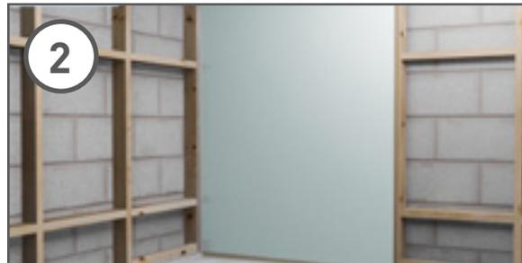
Bond the first panel to the wall or frame, with the grooved edge first. If screw fixing panels to the wall/frame, pilot bore the recess in the groove where screws are to be located. Failure to pilot bore may result in the panel's joint splitting). Pack between back of panel and wall as necessary to avoid distortion to the Hydrolock joint when screw fixing and to ensure that it is true and plumb.
