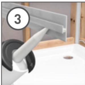
3 Apply silicone sealant to the channel of the second profile and attach it to the long edge of first panel.
