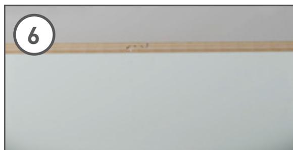
Remove the masking tape and ensure any excess silicone sealant is wiped from the laminate face immediately.
