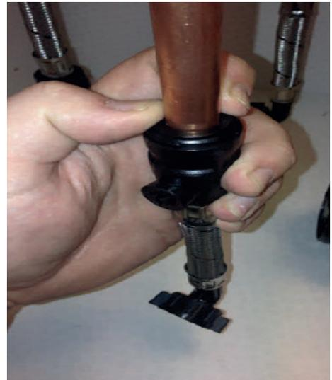
**6** The new pump can now be unpacked, the noise reducing rubber feet fitted and the pump offered up to the installation - if the installation will allow, the outlet flat washer can be fitted and the pump connected to the outlet pipework. If the installation will not allow this, the new, longer hoses may be used following the next steps...
