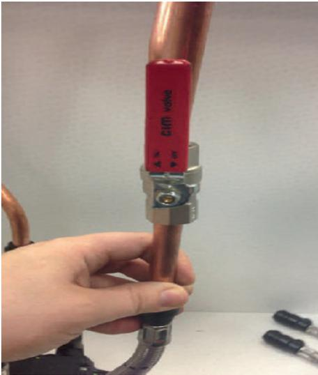
**10** Now, the water can be turned on, and you can check your connections for any leaks.
